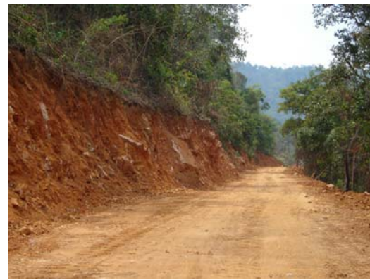
Current Renovated Road During Construction (April 2007)
